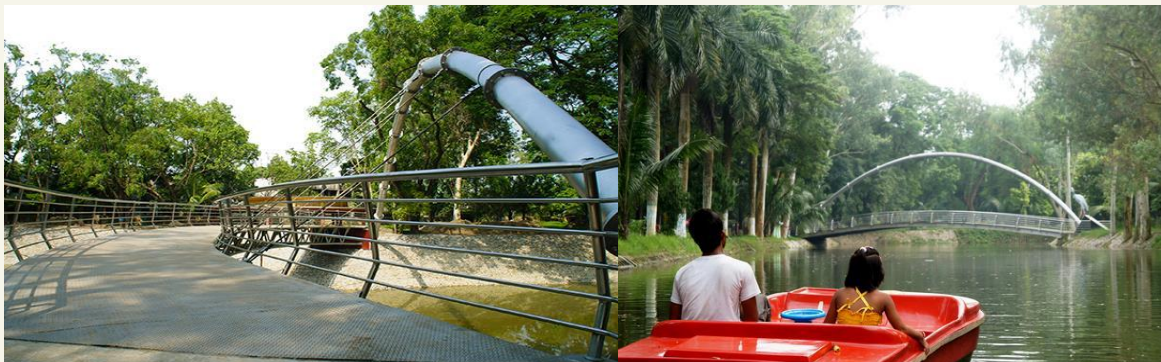
Construction of steel arch bridge having single span of 36m long bridge at Kamruzzaman Central Park at Rajshahi City Corporation, Rajshahi
