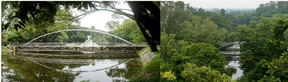
Construction of steel curve bridge 42m long integrated fixed supported bridge at Shaheed Kamruzzaman Central Park, KCP at Rajshahi City Corporation, Rajshahi
